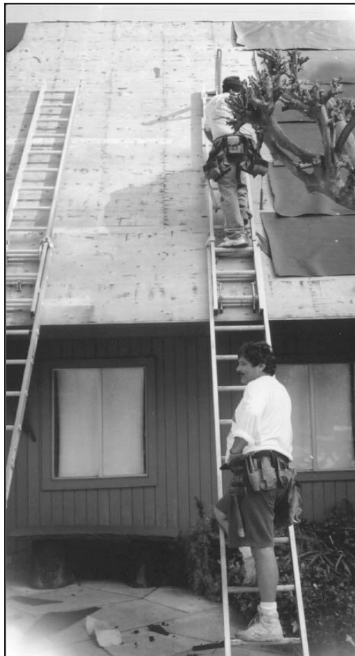
Our “Repair Fund” at work: Re-roofing the Chapel
